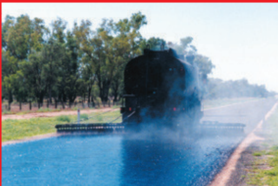
G Series Pumps provide high volume for rapid bitumen application.
